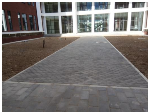
广场透水铺装 (2017.4)
